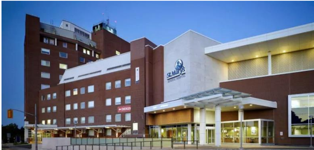
Figure 2. St. Mary's General Hospital
